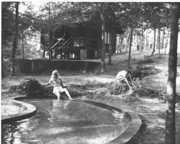
Cabin #4 and artesian well
